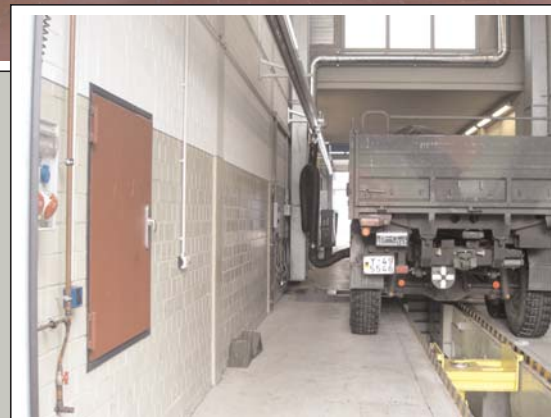
Rail system SSK 150 as travelling system at HGVs/LGVs brake test beds with single fan FD. Optional with automatic hose detachment from the exhaust and automatic return of the hose carriage via pulley drive.
