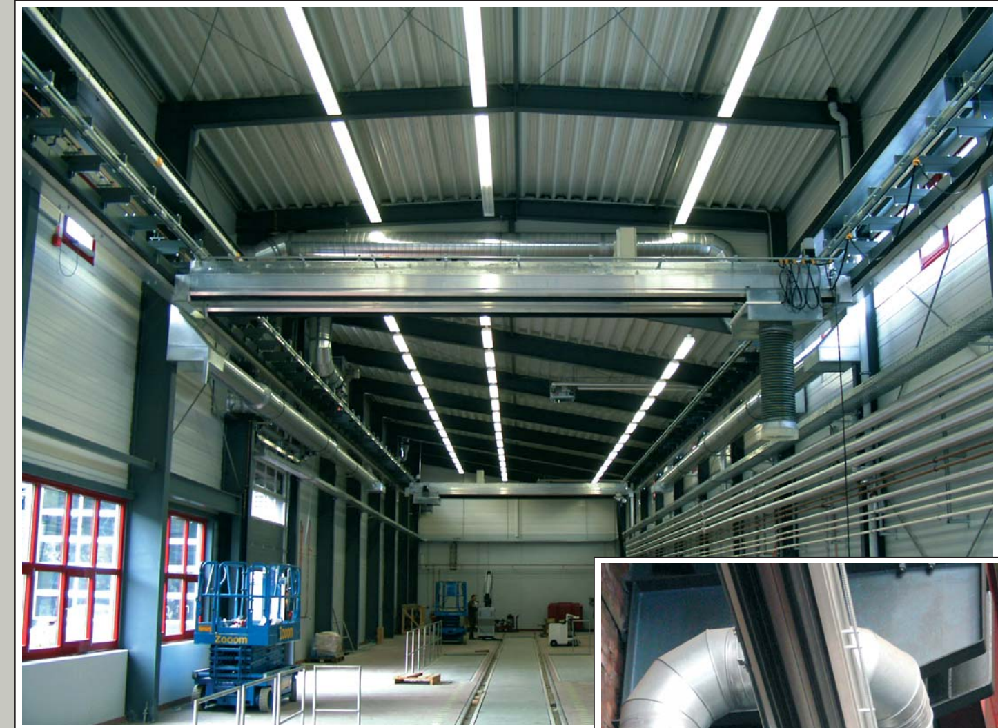
Rail system SSK 450 / SSK 900 as coordinate system movable with two extraction racks for diesel locomotive extraction with a free span of up to 12 m, movable lengthwise 60 m. The system is installed underneath a crane facility and both systems are locked against each other in accordance with safety regulations. Operation is electively via hand control or radio remote control. Possible suction performance of up to 20,000 m 3 /h.
